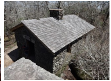
The shelter roof was replaced
