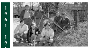
Road construction crew under Bud Akins at Tesnatee Gap, 1968
