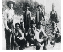
Local men build the road through Neel Gap
